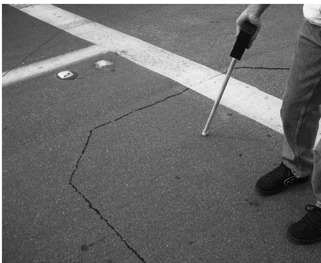
Left: Duane Dexter shows where to ideally place your tire for detection. If your tire is there, he figures your engine will be right over the loop detector's sensitive spots (right), causing the most disturbance in the magnetic field and tripping the detector.
